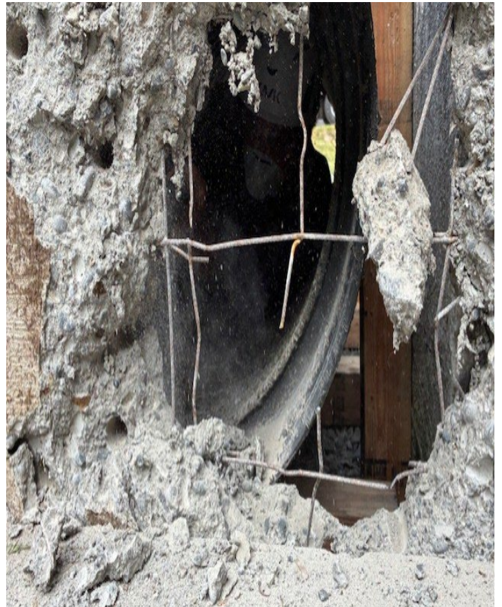
Laying in a restricted space cutting concrete
