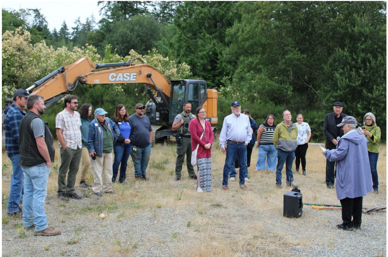
Groundbreaking ceremony on July 1, featuring attendees from Shold Excavating, Olycap, the Sheriff's Department, Jefferson County Commissioners/staff, the Warming Center and Bayside Housing. Photo by Rachael Nutting
