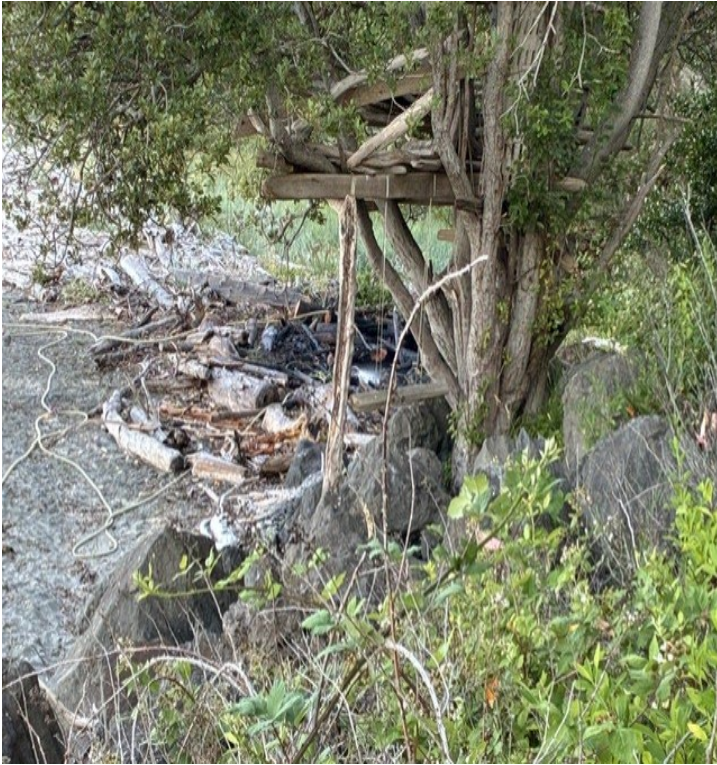
Driftwood Fire at Hood Canal Bridge
